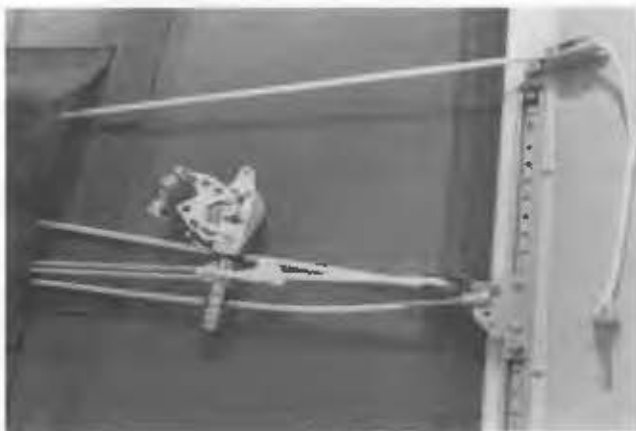
One side of 4-way system completed.
